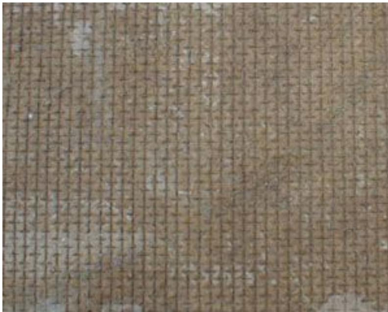
An example of the waffle Iron pattern for Masonite siding
